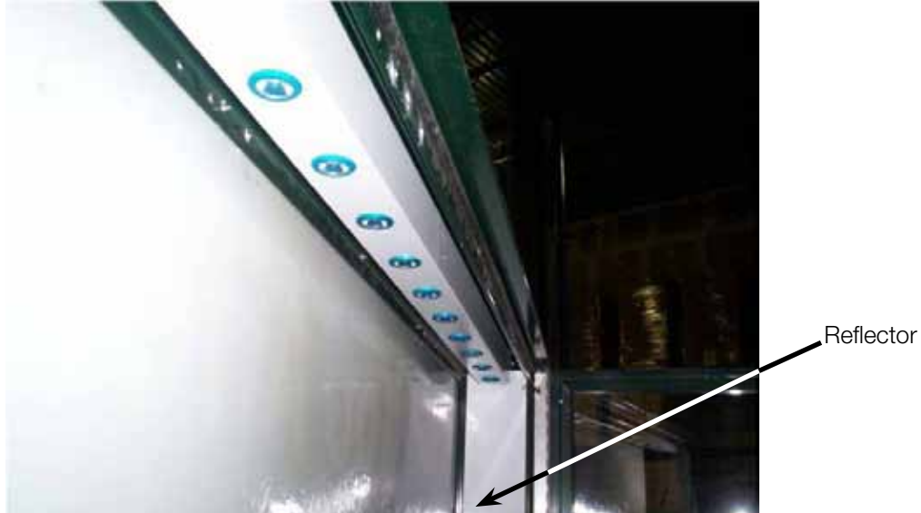
FIGURE 19 INSTALLING LED LIGHTBAR
