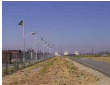
Fence and security lines
